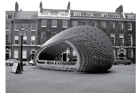
DRL pavilion in London: Complex assembly of interlocking planar parts (photo used under Creative Commons from jimmiehomeschoolmom)
