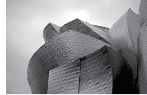
Guggenheim Museum, Bilbao: Complex geometric forms decomposed into developable surfaces (photo used under Creative Commons from Jaume d'Urgell)
